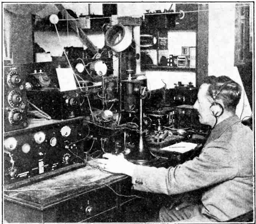
2ZG , owned and operated by Mr. W. J. Badman at 12, Southside, Weston-super-Mare, who is here seen at work on the 200 and 400 metre telephony transmitter. A Meissner circuit is employed; the output from the "Round" microphone is passed through the amplifier on the left to a choke modulator.
