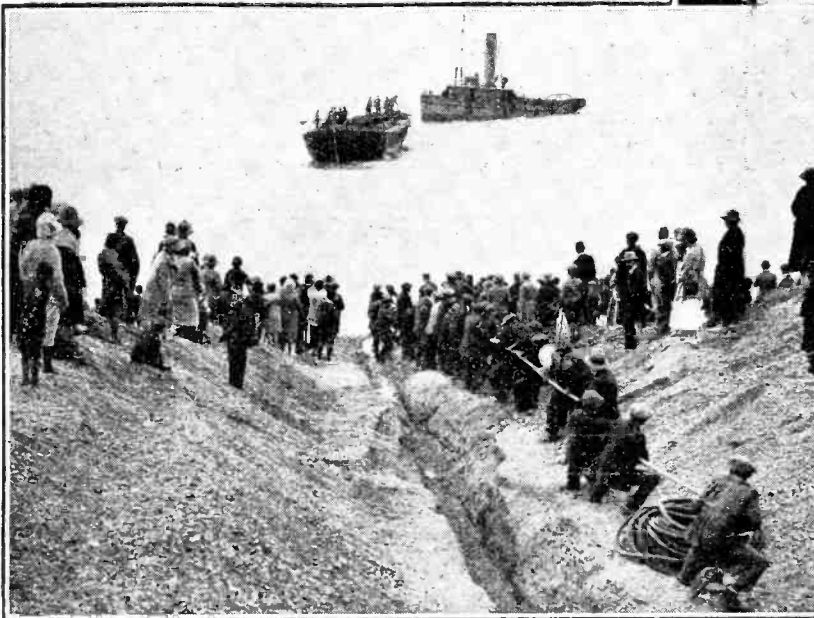
Landing and hauling ashore the end of a submarine cable. In this instance the weight of the cable is 25 tons to the mile.
