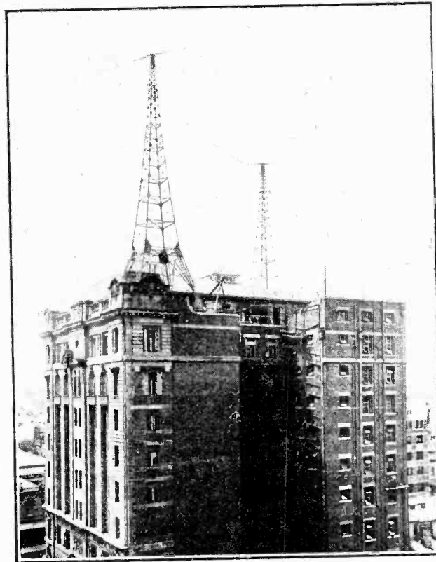
AUSTRALIA CALLING. 4QG, the broadcasting station at Brisbane, Queensland. The aerial system is erected on the highest building in the city.
