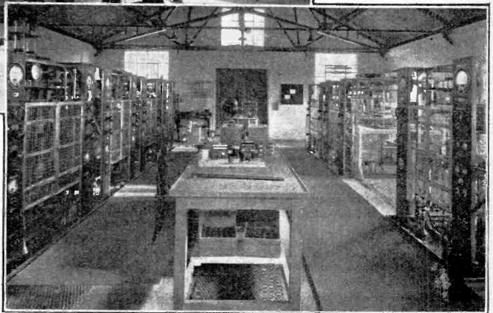
Lower charges combined with a fairly efficient service have attracted a considerable amount of traffic from the cables to the Empire beam wireless services. (Upper) The Bridgewater Beam Receiving Station built by Marconi's Wireless Telegraph Co., Ltd., for the General Post Office. There are two receivers for reception from South Africa and Canada. (Lower) The beam station transmitting room at Dorchester. The set on the left is used for communication with New York on three separate wavelengths, and the set on the right communicates with Rio de Janeiro.
